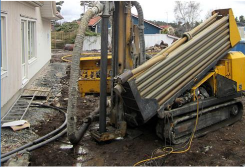
Thermal & Water Wells
