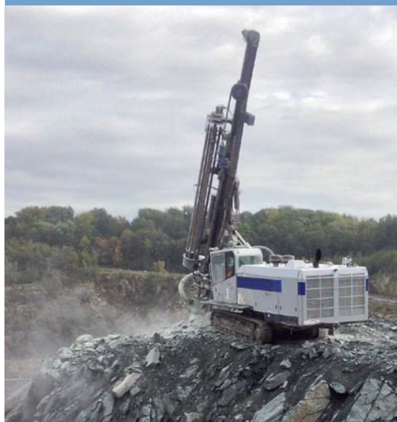
Quarry in Belgium – 4" BulrocRobit hammer in use.
