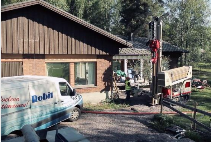
Thermal & Water Wells
